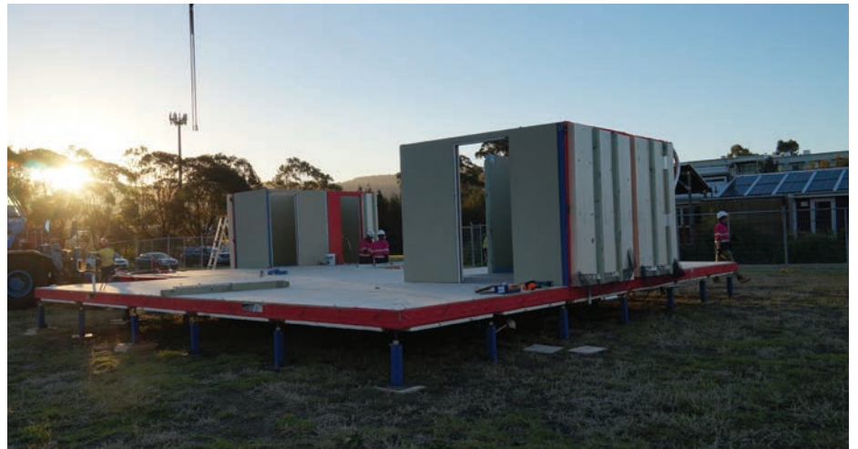
Figure 2.7 - Pods and Floors Assembled
