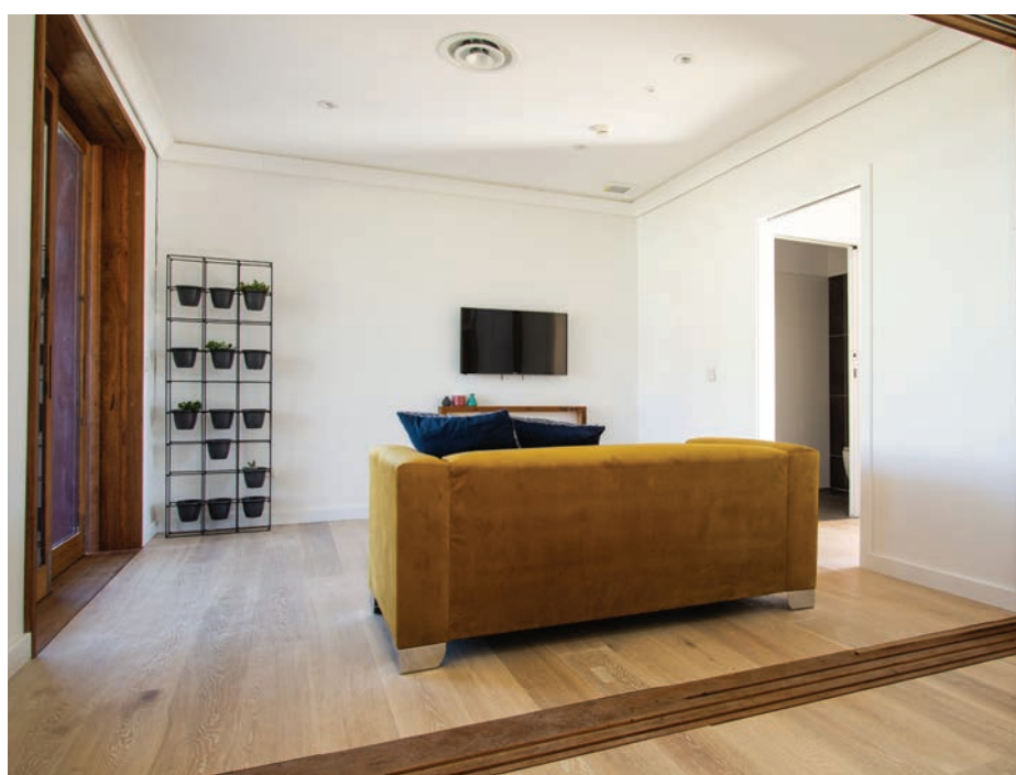
Figure 2.48 - Living Room Showing Sliding Wall Panel Track On Floor
