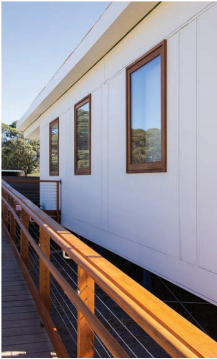
Figure 2.30 - Weathertex Cladding
