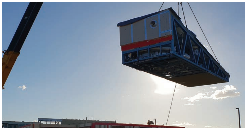
Figure 2.8 - Large HVAC Cage Being Lifted
