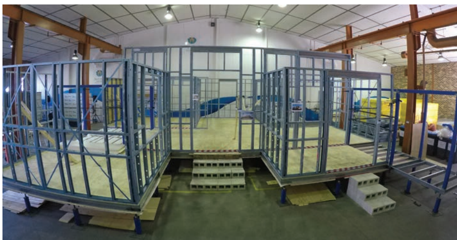
Figure 2.9 - Photo Taken of Structure
