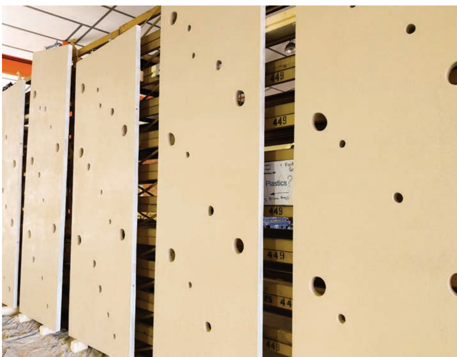
Figure 2.21 – Second Skin Wall Panels Freshly Painted
