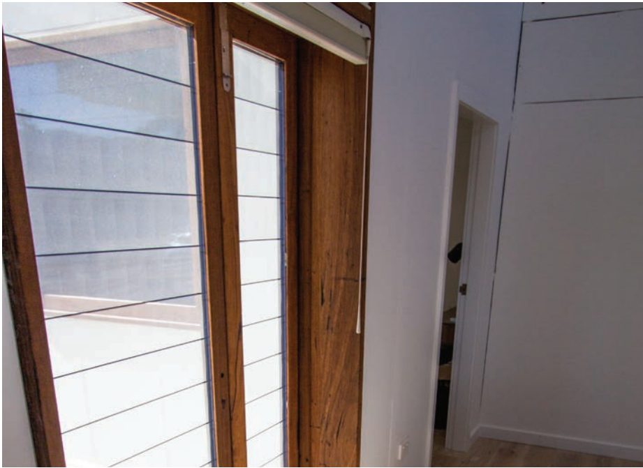
Figure 2.22 – Microshade Strips Visible on Doors on the South Facing Side of House
